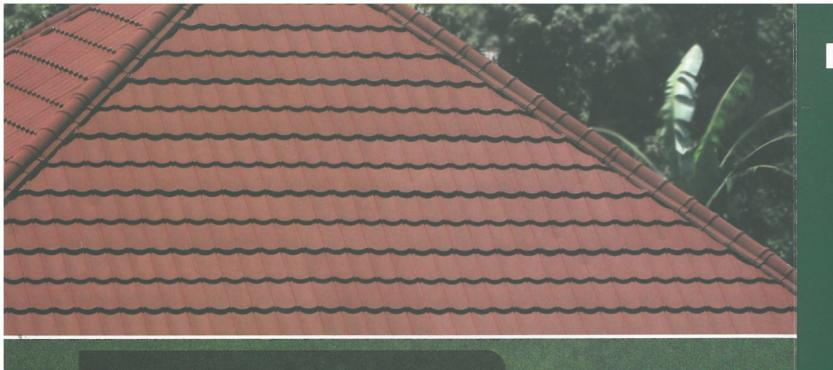
Metal tile MULTI ROOF, MULTI SIRAP and FANCY using stamping system with progressive dies that produce metal roof with beautiful shape and compact with high accuracy.
